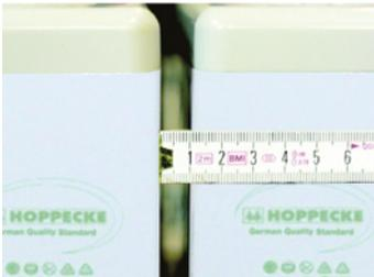
*Fig. 5-14: 10 mm clearance between the batteries*
